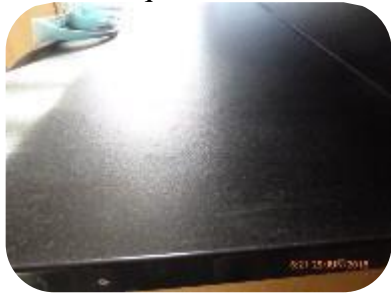
Requires to be cleaned
