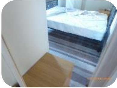
Requires to be cleaned
